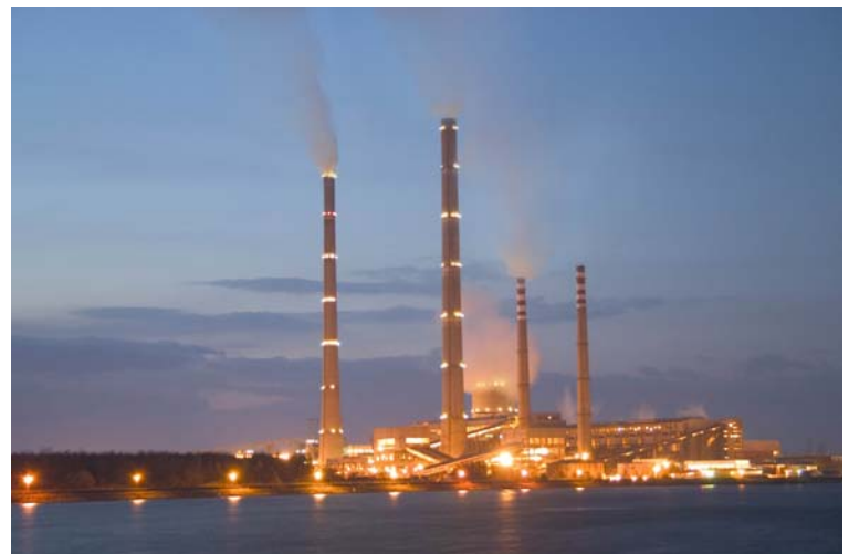
Honeywell modernized Maritsa East 2 and improved plant productivity.
