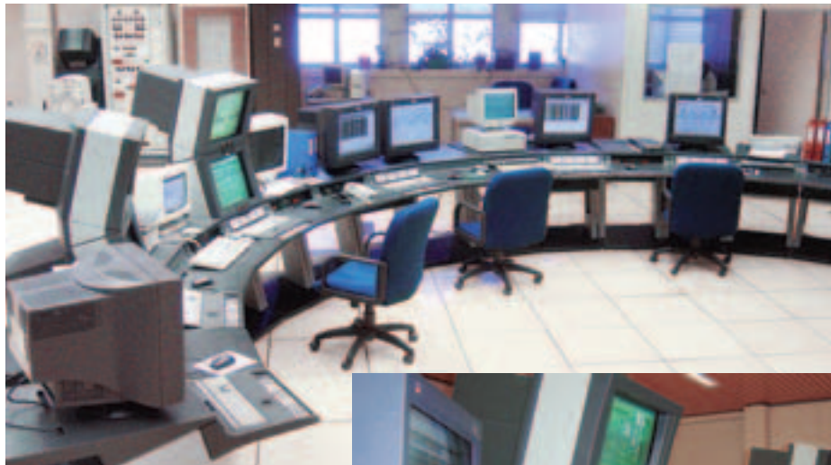
Display and alarm standardization was a key element. Since the human machine interfaces had been designed by ENSI's operators, most displays were highly populated, and their performance was less than ideal—although they were functional.
