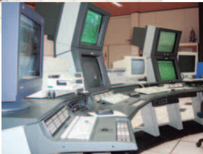
Display and alarm standardization was a key element. Since the human machine interfaces had been designed by ENSI's operators, most displays were highly populated, and their performance was less than ideal—although they were functional.
