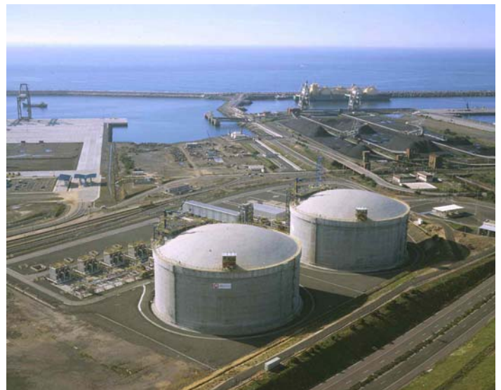
Transgas Atlantico’s Sines LNG terminal implemented Honeywell automation solutions for continuous safe and reliable operations.
