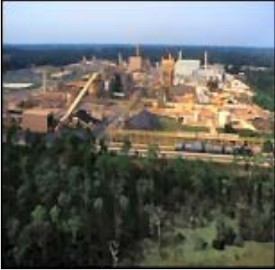
Figure 2. DuPont's DeLisle TiO 2 plant
