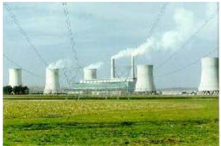
Honeywell’s advanced alarm management solution has helped the Grootvlei power station to manage alarms more effectively.
