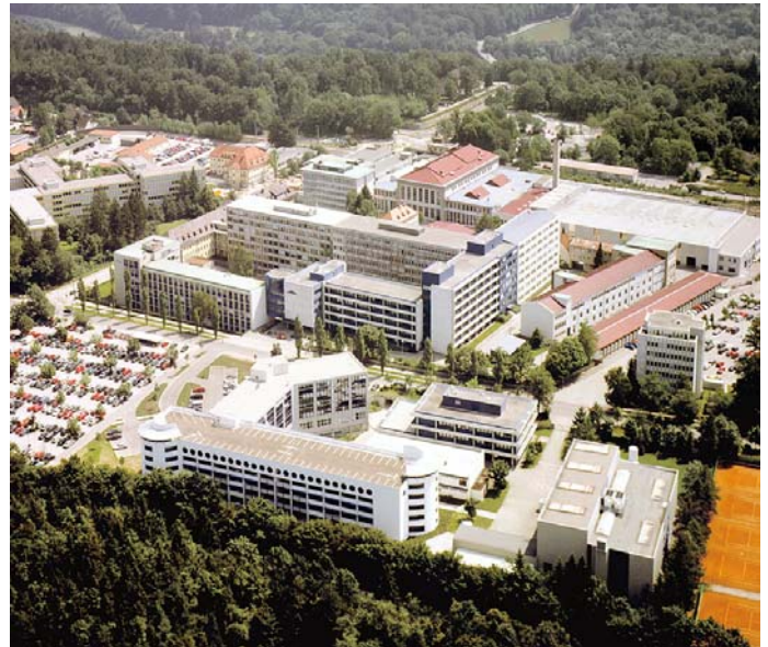
Linde Engineering chose to migrate to Honeywell's UniSim simulation software for olefin, hydrogen and synthesis gas plants
