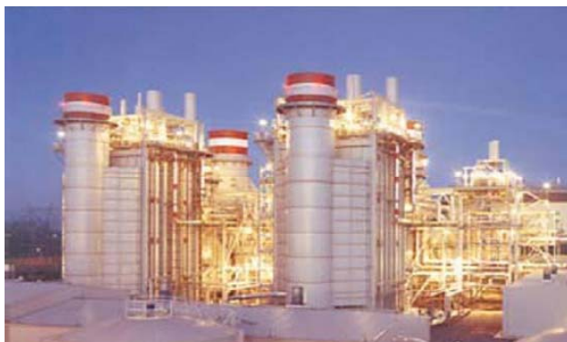
Figure 1: Industrial Power Plant
