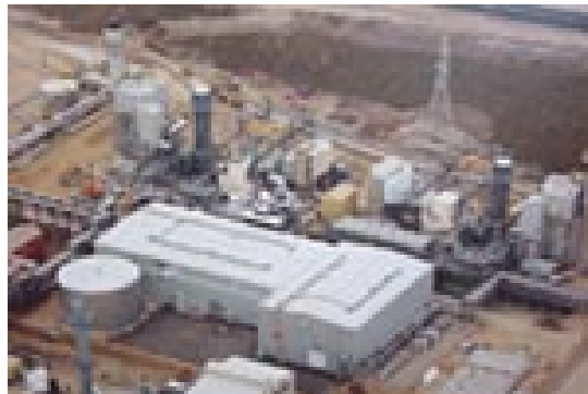
TransAlta's Poplar Creek facility relies on Honeywell simulation technology for onsite training and testing.
