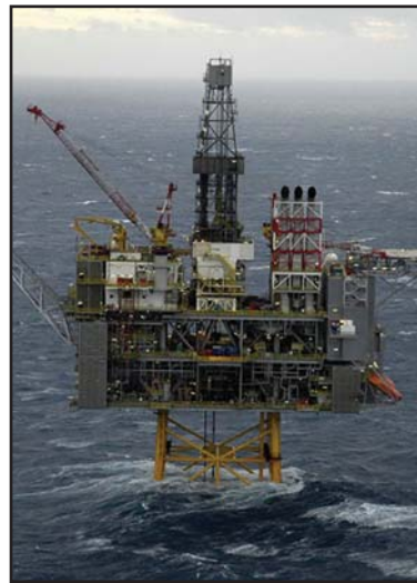
Honeywell installed an integrated control and safety system for British Petroleum's Clair offshore platform.
