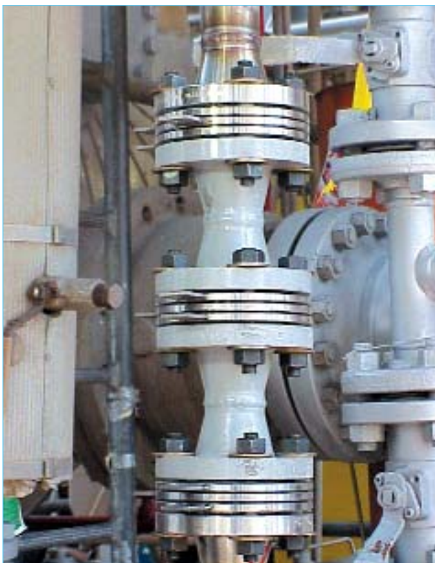
Figure 3. Installation of carbon steel, 304L, and 316L probes in 8 in. pipeline.
